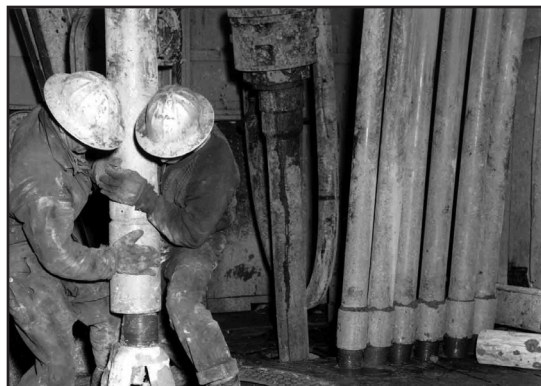
Fig. 3 These two roughnecks are changing a rock bit on a Shell rig, some time in the late 1950s. Photo courtesy Shell Canada Ltd.
