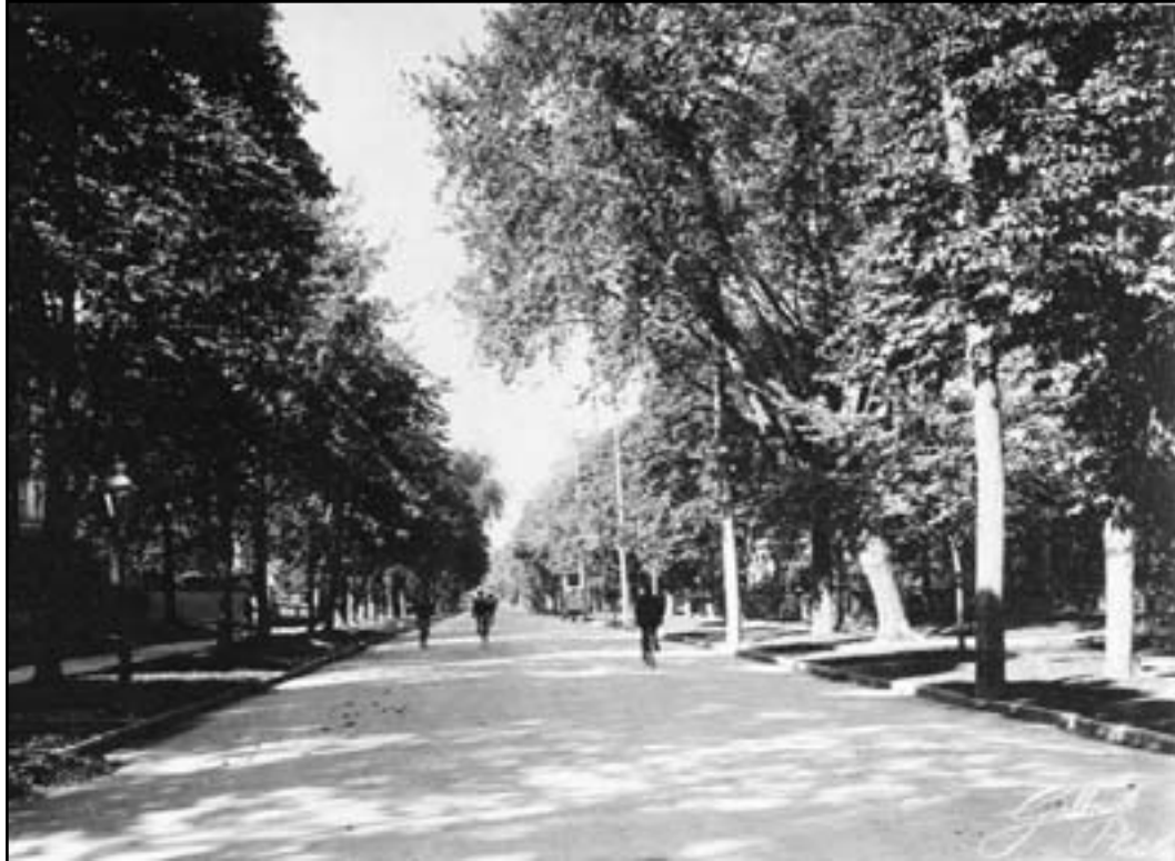
Fig. 2 A properly paved environment (Permission Mike Filey)
