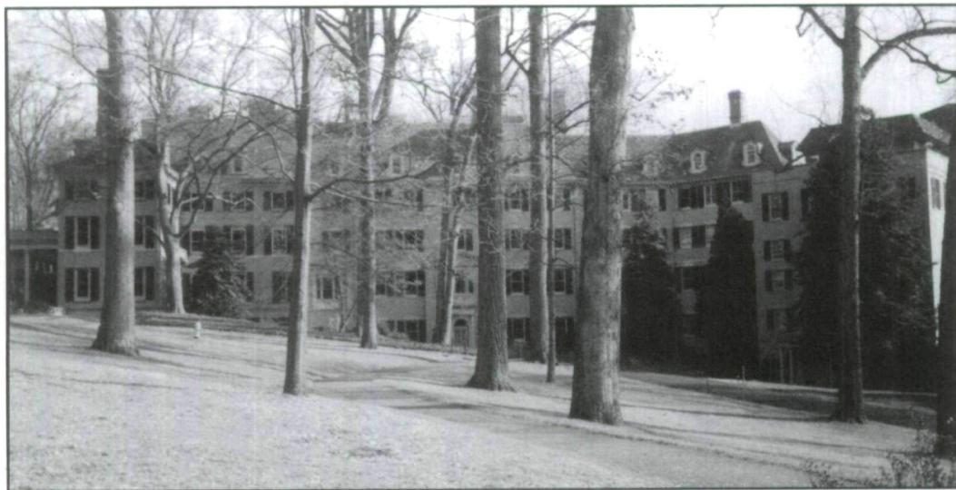
Fig. 1 The Winterthur Museum is located in Wilmington, Delaware.
