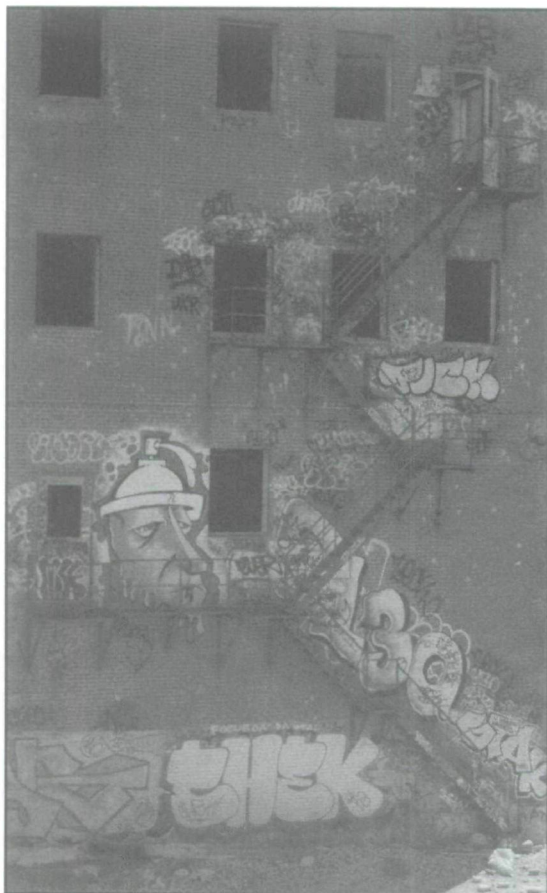
Fig. 1 Redpath warehouse on the Lachine Canal in Montreal, 1995.
