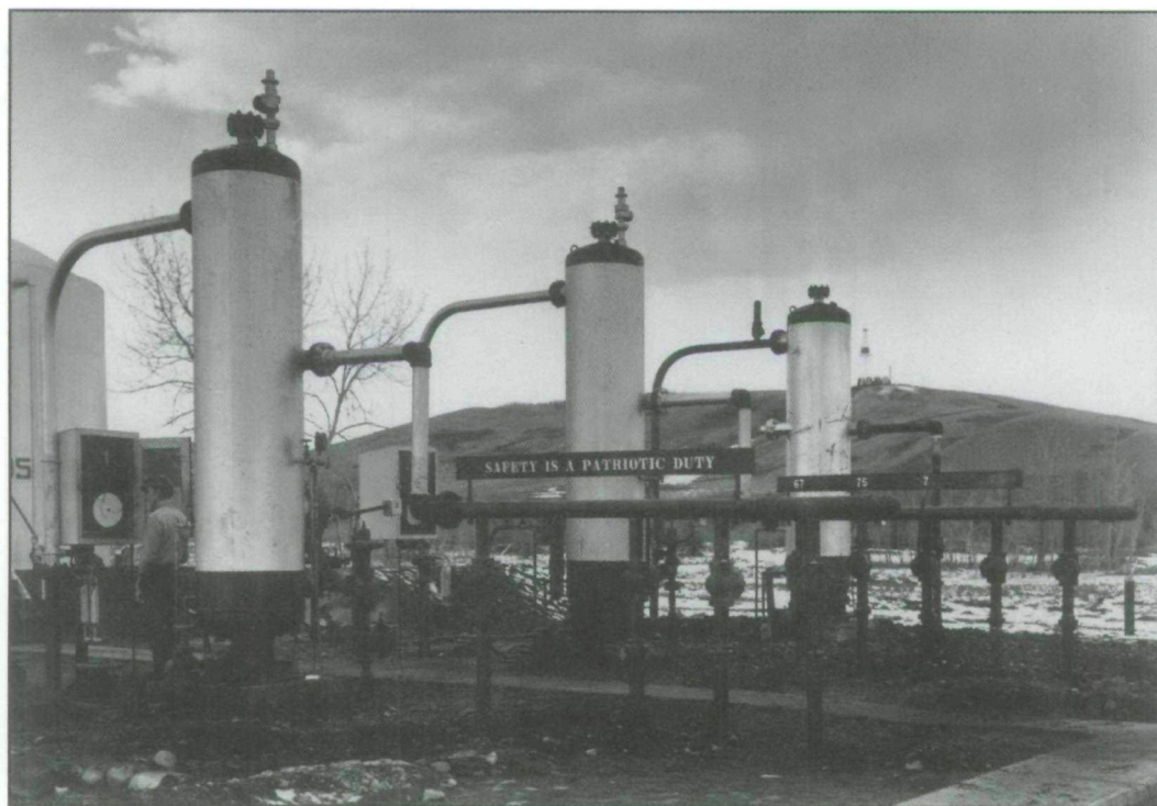
Fig. 1 During World War II, the plant functioned as a vital cog in the Canadian government's war machine and safety, as the sign says, became a patriotic duty. (Courtesy Provincial Archives of Alberta, Pollard Collection, P. 2384)
