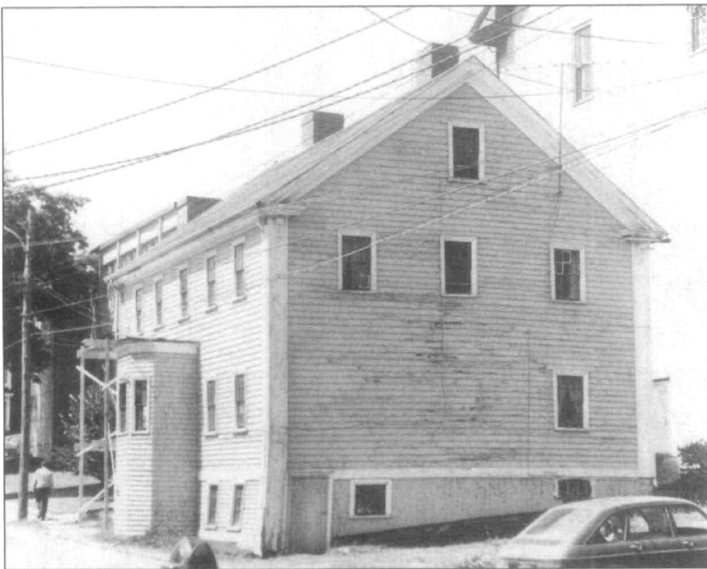
Fig. 2 The exterior of the Knaut-Rhuland house before removal of the turret-like "bump" in 1979–1980. (Photographer unknown)
