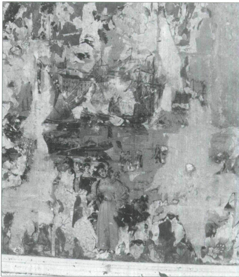
▲ Fig. 6 This was the best preserved piece of original scenic wallpaper found in the parlour. Although it was found throughout the room, some of it appeared to have already been removed, perhaps when the second layer of wallpaper was applied. The scene is printed in black, grey, and white with a repeat of 59 1/2 inches (151 centimetres).
