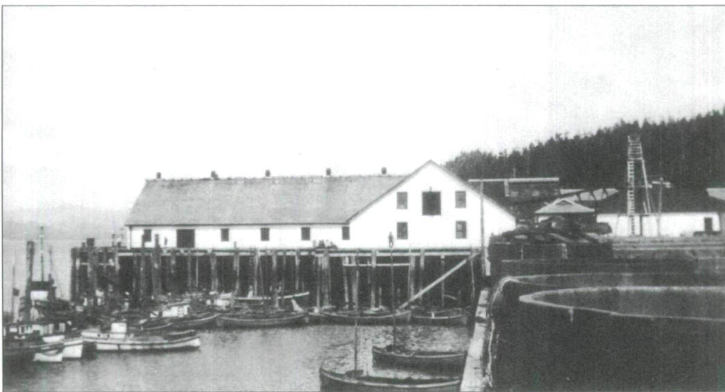
Fig. 3 Claxton cannery (Skeena River), 1928. Two fire protection measures are visible here: water barrels on the roof of the main canning plant and a watch tower to the rear. (Photo courtesy of Gordon Stead, Vancouver)
