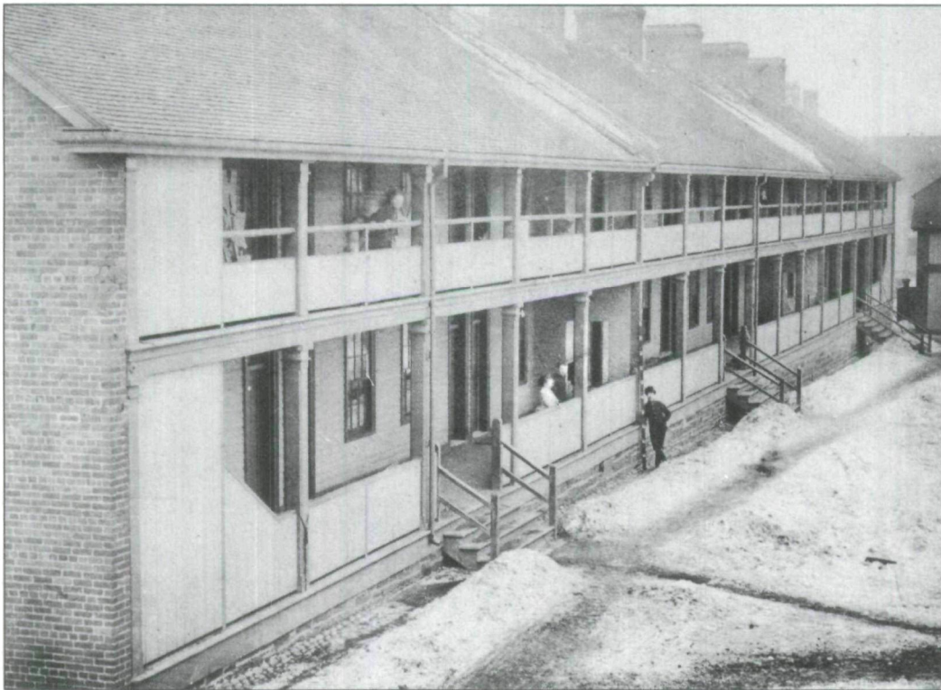
Fig. 1 Pavilion Married Quarters (southwest corner of Brunswick and Cogswell Streets) circa 1876. This building, for married non-commissioned officers and men, was built in 1867–68. Storm sashes do not seem to have been deemed a requirement. (Crown copyright photograph courtesy Controller of Her Majesty's Stationery Office, Public Record Office, WO 78/2835, London)
