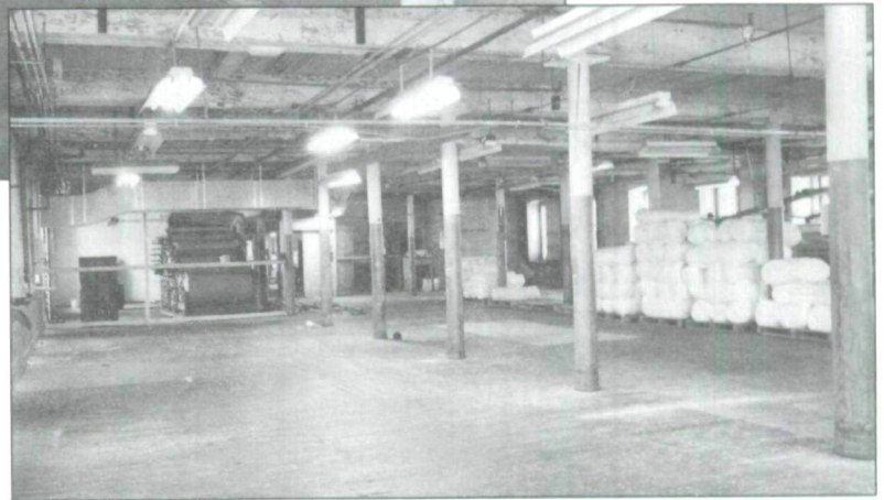
▲ Fig. 6 Slow-burning construction in the south wing of the Rosamond mill. (Courtesy: Canadian Parks Service, Canadian Heritage Recording Services)
