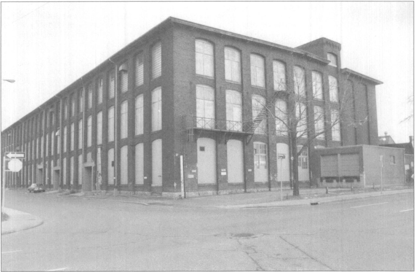
▲ Fig. 13 The Imperial mill in Hamilton (built 1900) shows the extent of window area possible in mills constructed on slow-burning principles. (Courtesy: Canadian Parks Service)
