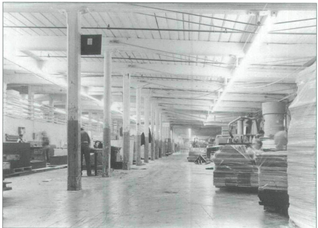
▲ Fig. 11 Interior of the reinforced concrete extension of the No. 1 mill. Note the increased window area. (Courtesy: Canadian Parks Service, Canadian Heritage Recording Services)
