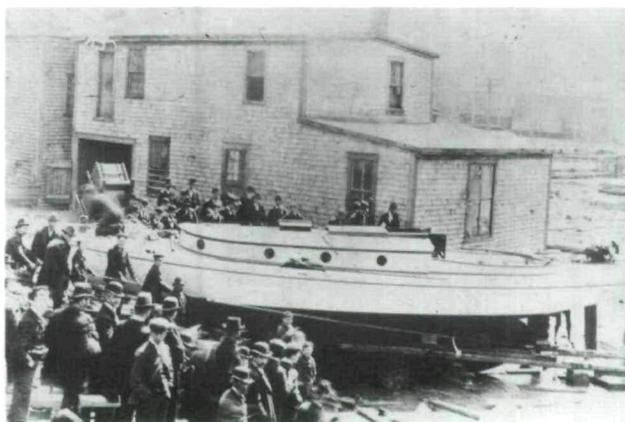
Fig. 2. The *Canada* being launched from the Hilyard boat yard, Saint John, New Brunswick, in 1898. Designed by Robert MacIntyre of Boston. Overall length: 42 feet; beam: 11 feet; registered net tons: 8.45; sail area: 1753 square feet. (Courtesy: New Brunswick Museum; from the collection of Col. G.G.K. Holder.)
