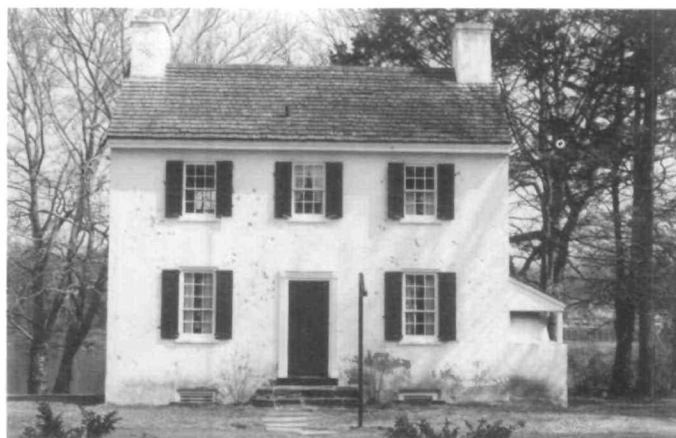
Fig. 3. Abdon Hibbs house, Washington Crossing (formerly Taylorsville), Bucks County, Pennsylvania, built c. 1820 and restored by the Pennsylvania Historical and Museum Commission. A common house type in late eighteenth and early nineteenth century Bucks County. (Unless otherwise specified, this and subsequent photographs are by the author, March 1984.)
