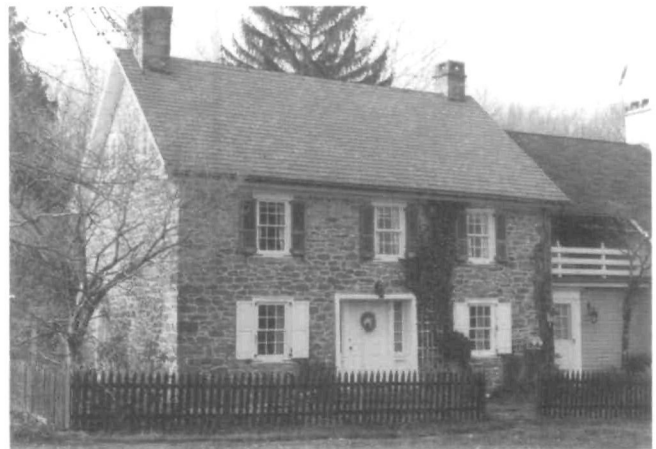
Fig. 5. Three-room-plan stone house, surrounded by lands owned in the late eighteenth and early nineteenth centuries by Ebenezer, John, and Joseph Doan, Phillips Mill Road, just outside the village of Solebury, Bucks County. Recent additions have been made to the side and rear of the house, while the front doorway was enlarged and sidelights were added probably in the mid-nineteenth century. (April 1984)
