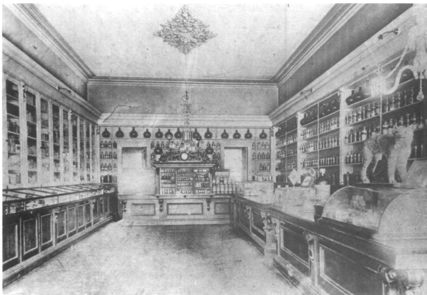
Fig. 2. The earliest interior view of the Niagara Apothecary (then Randall's), about 1900-1910. Most of the crystal drops had already been removed from the original Confederation-period gasoliers, at first fuelled by gas manufactured on the premises, but by this time converted to electricity, as were extra wall fixtures on either side. The elaborate plaster bas-reliefs in the ceiling were untouched and remain to the present day. (The original light fixtures still hang too, but unfortunately in private homes elsewhere in town, with careful replicas replacing them in the shop.) The prescription counter at the back centre is surprisingly small, considering that most dispensing at the time consisted of preparing prescriptions "from scratch," before the shift to large-scale manufacturers. Witness all the containers that ranged the shelves across the back and along the right side of the shop. They and the bins and drawers below, not to mention carboys, barrels, drums, and crocks in the back room and below, carried raw materials in various stages of preparation from crude to semi-finished. By the time this photo was taken, the original prescription counter (centre section) had been extended on either side (on the left ultimately to house a postal substation). Otherwise, the fixtures of solid black walnut and butternut installed in 1866 remain to this day. Shelves and glass-topped cases along the left side and the countertop cases at right carried proprietary or patent remedies, toiletries, and sundries. (Collection of the Niagara Apothecary; photographer unknown.)
