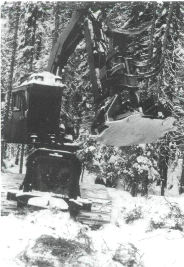
Fig. 10. Crawler-type tree harvester with hydraulic-powered arm and felling head, ca. 1978. (Photo: private collection.)
