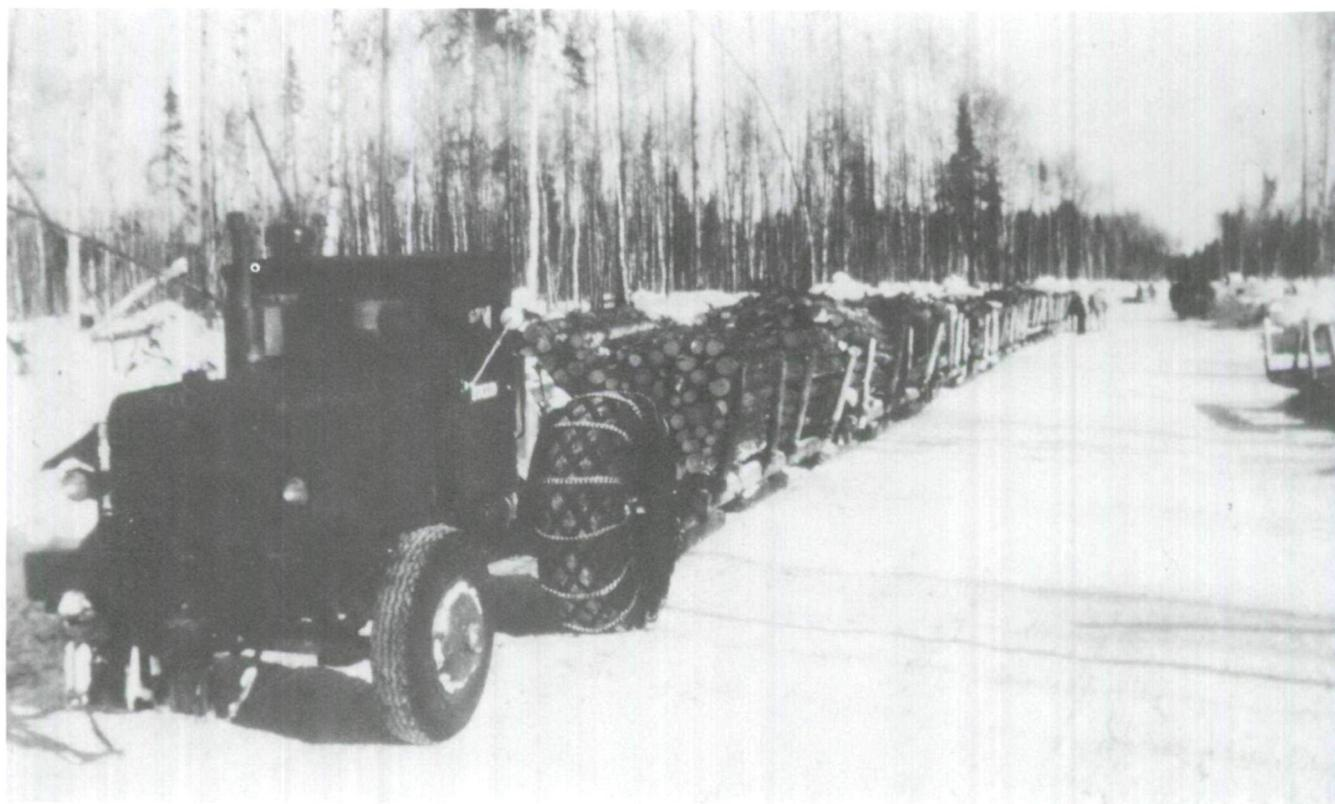
Fig. 5. Euclid 200-horsepower diesel truck pulling ten sleighs loaded with eight-foot pulpwood at Nipigon Lake Timber Company Camp 71, near Kowash, Ontario, 1948. (Photo: University of Toronto Archives, A73-0025, Logging Report by W.E. Cuff, 1948.)
