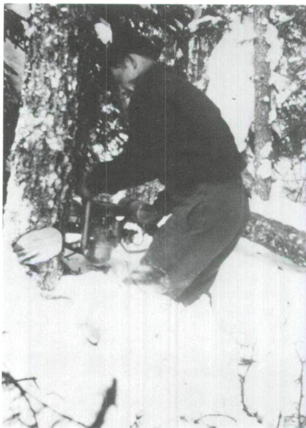
Fig. 7. Felling with an early model chainsaw that weighed over fifty pounds. The Kormak Lumber Company employee pictured here found the saw heavy and prone to breakdowns in 1948. (Photo: University of Toronto Archives, A73-0025, Logging Report by K.G. Crowhurst, 1948-49.)
