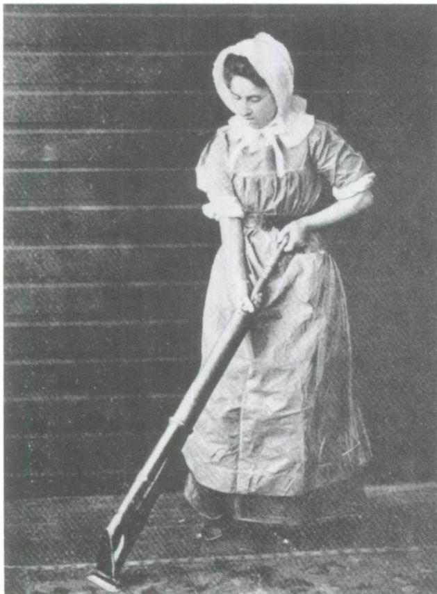
Fig. 14. Working the vacuum cleaner. The right hand slides one metal type up and down another, operating a small air pump whose sucking power is testified to by "a head of the finest grey powder." (Alice Ravenhill, "Labour-Saving Devices in the Household," *Bulletin* no. 41, British Columbia Department of Agriculture, [1912], p. 17.)
