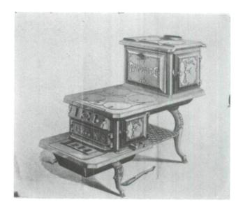
Fig. 7. Favourite cook stove (with elevated oven) burning coal or wood, with a "shaking, dumping and clinkerless" ash pit, registered by James Moffit Spencer of Nova Scotia, 1877. Vol. 77. (PAC, RG105.)
