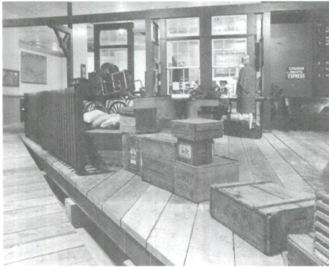
Fig. 4. Reconstruction of a typical western CPR station, 1930. (Photo: Ron Marsh, Glenbow Museum P2594-219.)
