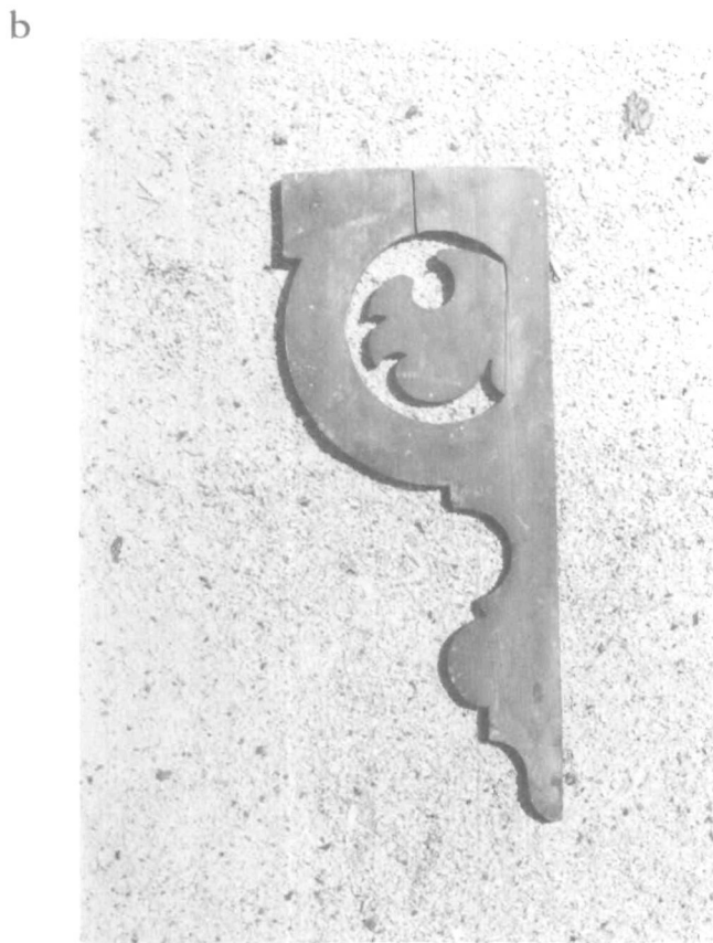
Fig. 2. Bracket patterns at the Sutherland Steam Mill: a, length 44 cm, width 23 cm; b, length 49 cm, width 20½ cm; c, length 25 cm, width 14½ cm; d, length 32 cm, width 15 cm. (Photos by the author, uncatalogued.)
