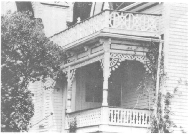
Fig. 6. Detail of verandah on Alexander Sutherland House showing decorative elements produced at the Sutherland Steam Mill. (Photo by the author, uncatalogued.)
