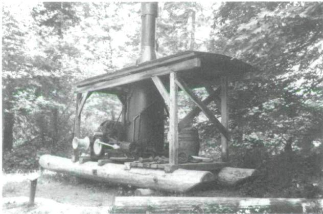
Fig. 2. Donkey engine, manufactured by the Victoria Machinery Depot, on display at the British Columbia Forest Museum. (Photo: British Columbia Forest Service [B.C.F.S.], neg. no. 21517/1.)
