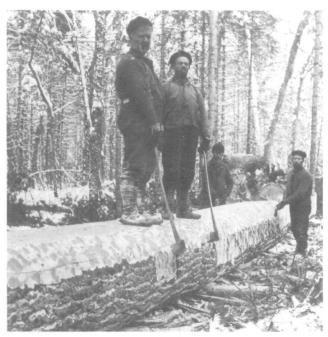
Fig. 7. The scorers moved ahead, notching the timber to the appropriate depth. The hewer followed, using the broad axe to produce a flat surface. (Photo: PAC, neg. no. PA-121800.)
