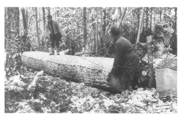
Fig. 6. The liner pulled the chalk line taut and let it snap against the timber, marking a line which was used by scorers and hewers to complete squaring the timber. (Photo: PAC, neg. no. PA-121801.)
