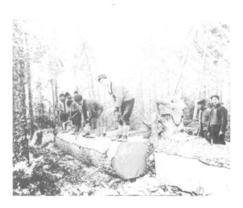
Fig. 5. "Rossing" or removing the bark from a piece of timber in preparation for the chalk line. (Photo: PAC, neg. no. PA-121797.)
