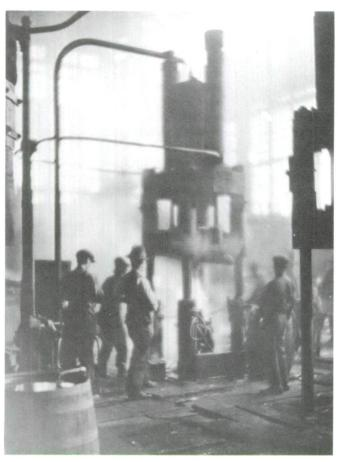
Fig. 11. Forging core of 75mm shells, Ellis Chalmers Company, Toronto, attributed to Pringle and Booth, 1914-1918. (Public Archives of Canada, neg. no. C-3193.)
