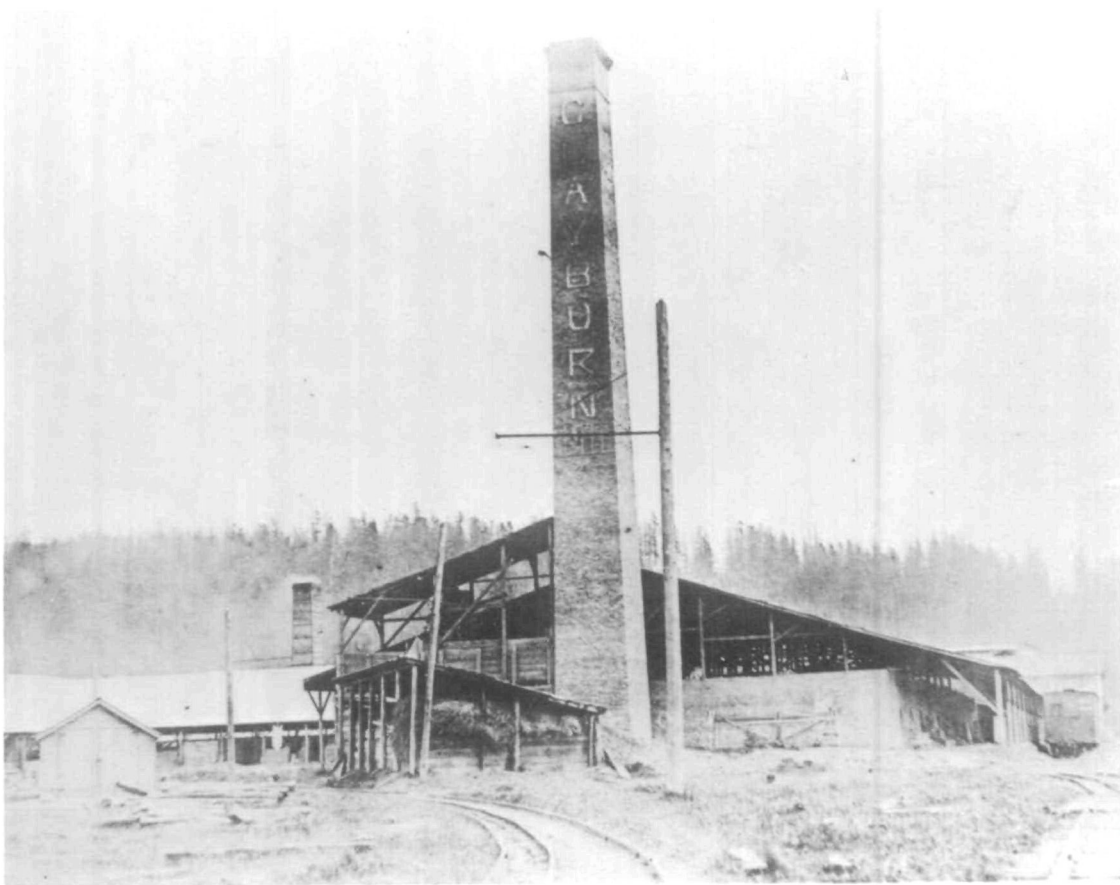
Fig. 8. A landmark on Matsqui Prairie after 1911, this smokestack for a continuous kiln bore the name "CLAYBURN 1911" in raised brick on one face. Demolished ca. 1930. (Photo ca. 1919; private collection.)
