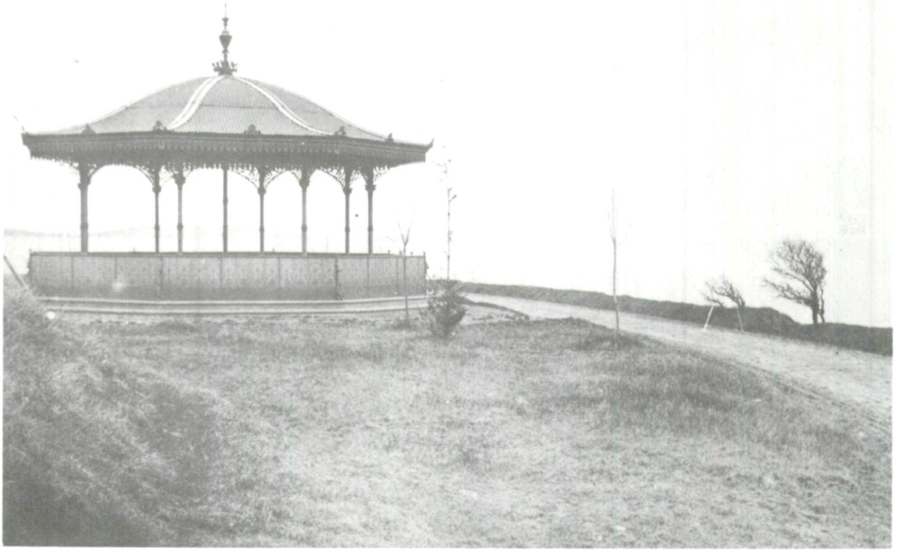
Fig. 1. One of two identical pavilions in Point Pleasant Park, ca. 1890, made by Macfarlane and Company, Glasgow, Scotland. The columns and brackets are cast iron and the roof is corrugated iron. (Photograph by Nova Scotia Museum, neg. no. 7412.)
