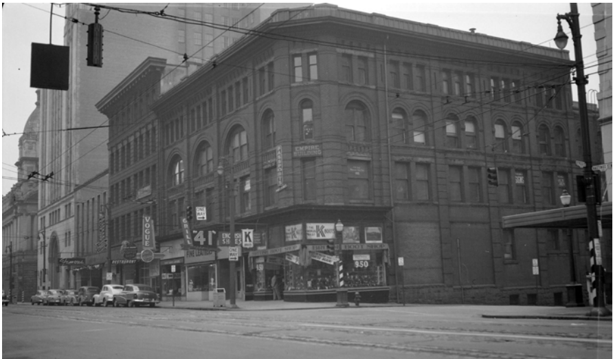
Fig. 1. Davis Chambers Building (c. 1955), 615 West Hastings at Seymour, Vancouver. (Photo credit: City of Vancouver Archives, CVA 447-329, photographer Walter E. Frost.)
