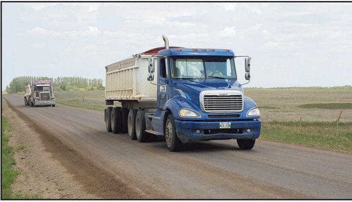
Figure 2. Curries Landing haul road near Brandon, Manitoba after stabilization using clay-rich soil and organic catalysts. Photo: Cypher Environmental.
