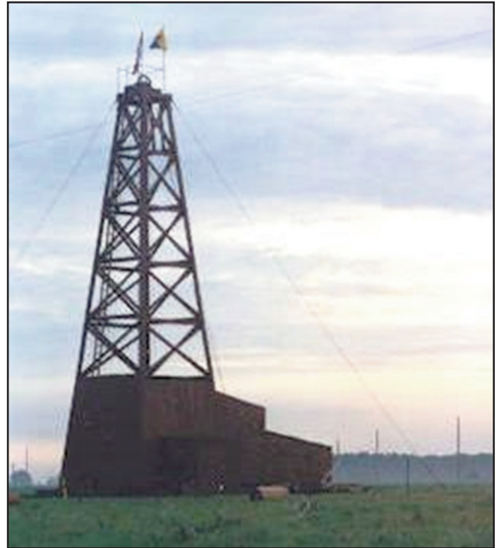
Figure 3. Canadian Drilling System rig rebuilt in 1996.
