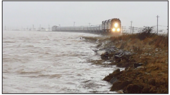
Figure 13. CN railway at Tantramar marshes on the New Brunswick–Nova Scotia border during high tide with storm surge of 60 cm, November 2015. Wave splash reached the rails. Photo by Mike Johnson, Cumberland Regional Emergency Management, reproduced with permission.
