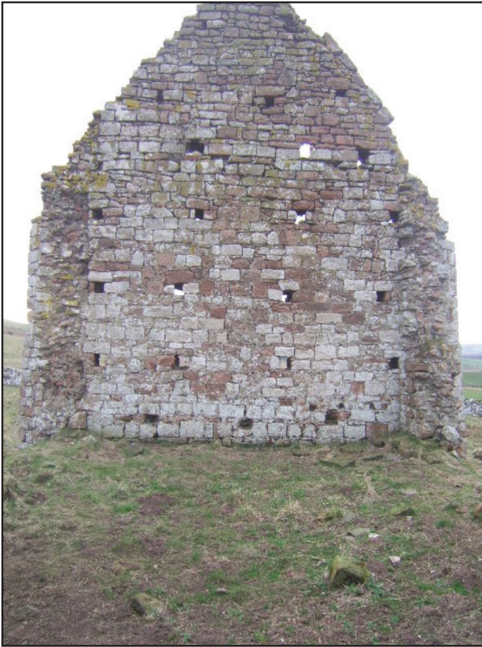
Plate 3. The ruins of St. Helen's Chapel, which the trail passes. Note the mixture of red and grey-green stone blocks used in construction.
