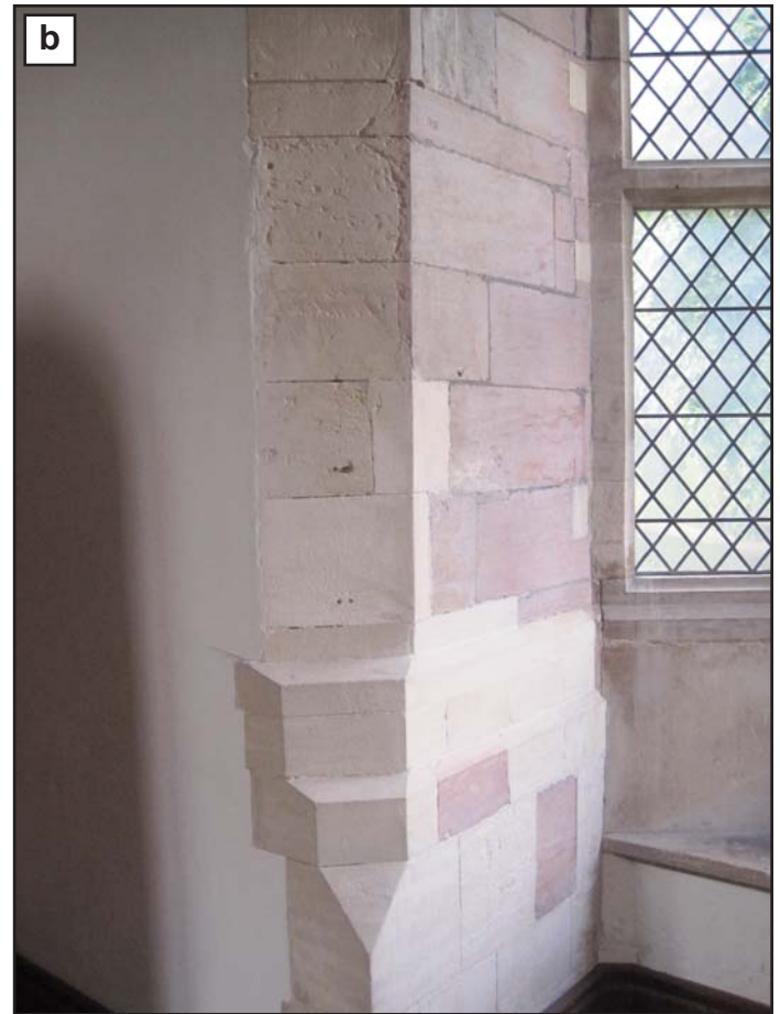
Figure 4. Examples of controversial or poor practices of stone usage. a) Queen Elizabeth II Courtyard, British Museum, London; b) contrasting replacement of stone in the interior of the Lincoln Cathedral, and c) replacement with stone of a different colour disrupting the original colour pattern in the exterior of the cathedral, Chipping Norton, Oxfordshire.
