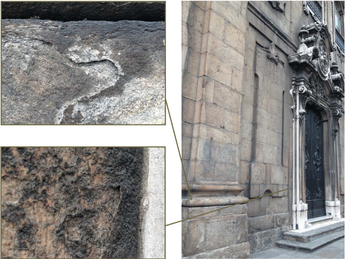
Figure 8. Degradation observed in historical buildings and identified as black crust. Formed by the accumulation of particles deposited on the flat surface of fine-grained garnet gneiss, the crust is associated with a blistering process on the façade of the Carmelite church, Rio de Janeiro.
