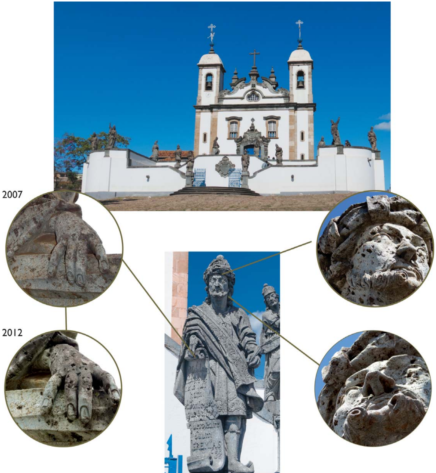
Figure 6. Deterioration of steatite (soapstone) works produced in the late 18 th century, such as those shown here in Congonhas Sanctuary, mainly caused by weak rock resistance, and by biological and anthropological factors leading to cavity or alveoli formation.
