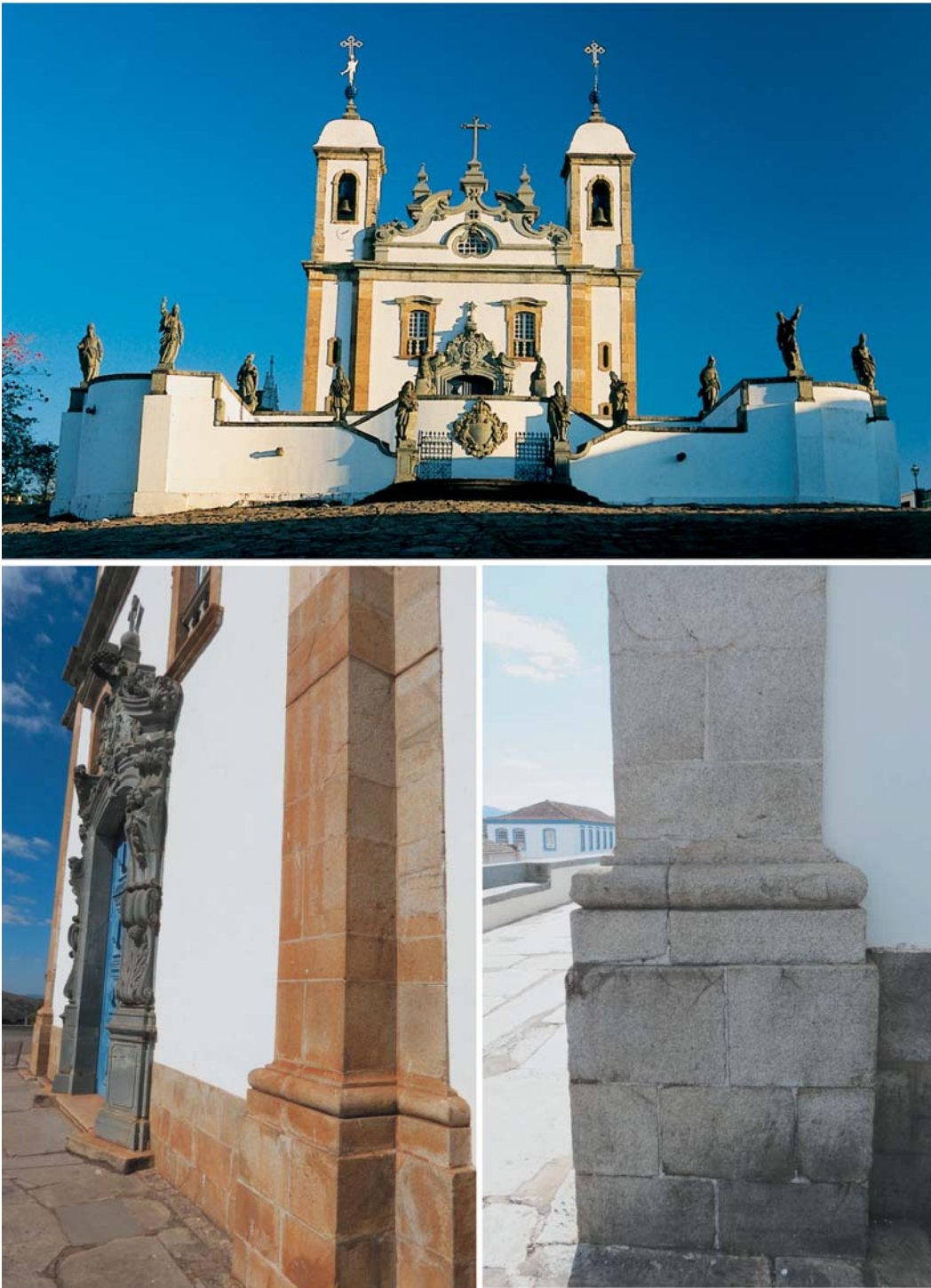
Figure 7. Example of patina formation (oxidation), deposition of particles, and biological colonization on the surface of granite blocks with whitish-grey original colour, on the frontispiece of the Congonhas Sanctuary of Bom Jesus church. The current brownish colour (patina) results from the position of these (outer) blocks facing the action of wind currents and variations in moisture content. In areas unaffected by such currents, the granite retains its original whitish-grey colour, although it is susceptible to intense biological colonization.
