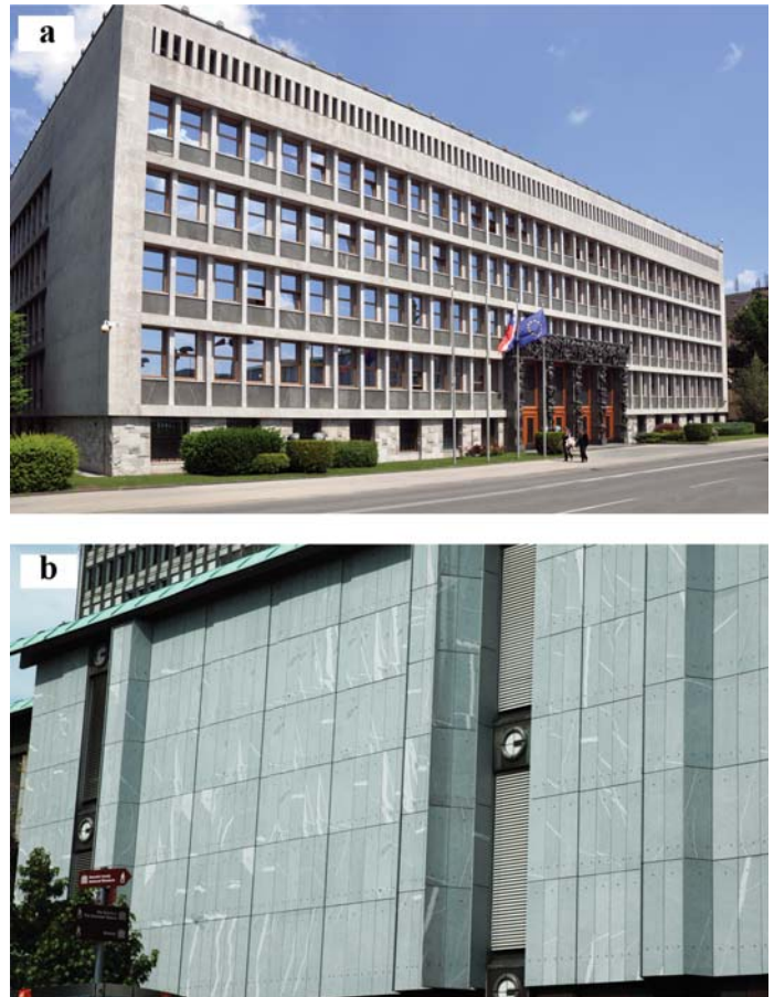
Figure 10. a) Granodiorite is used in the staircase of the Slovenian Parliament. Dark grey panels of the façade are made of cizlakite. Photo: Matjaž Zupanc. b) Maximarket department store with granodiorite façade. Photo: Miran Udovč.
