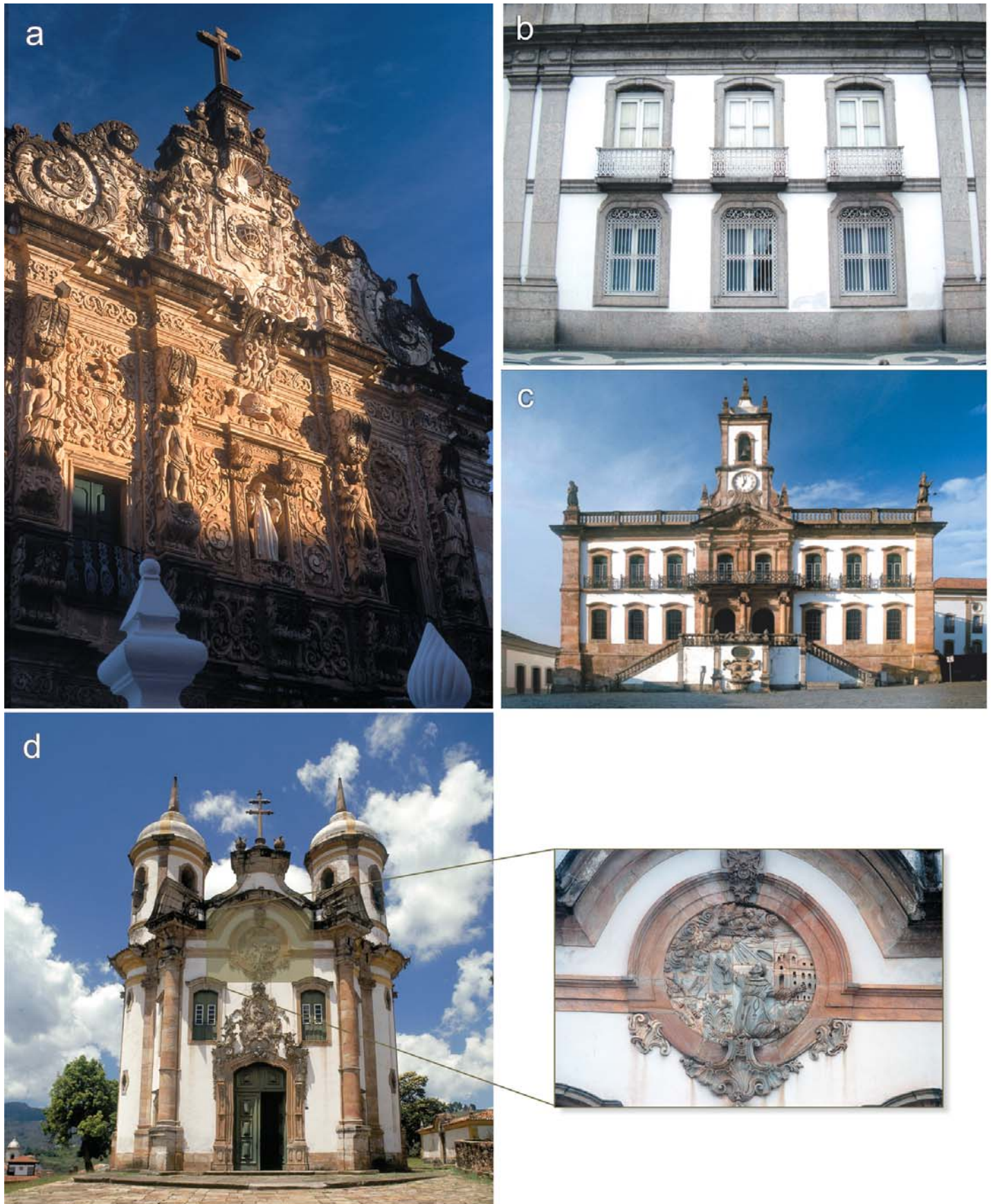
Figure 2. Selected uses of stone in the construction of Brazil's cultural built heritage. a) Limestone and sandstone in the frontispiece at the Chapel of The Third Order of Saint Francis, Salvador, Bahia; b) gneiss in a building in the city of Rio de Janeiro; c) quartzite in the old Casa de Câmara e Cadeia (Chamber and Prison House), located in Ouro Preto; and d) quartzite and steatite in the frontispiece of the Chapel of The Third Order of Saint Francis, Ouro Preto, Minas Gerais.
