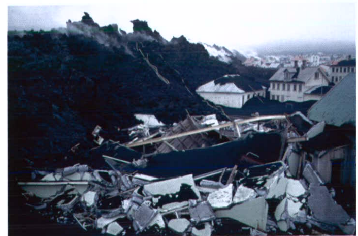
Figure 5 The lava advance into the town destroyed several hundred buildings including reinforced concrete structures in the harbour area. Cooling hoses can be seen on the lava front in the centre of the photograph.
