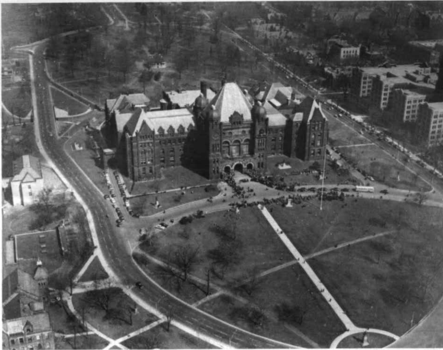
Figure 10 View of Queens Park looking north showing the fourth floor and dormers added by E.J. Lennox to the West Wing of the Parliament Buildings. This addition temporarily met the need for extra office space, but altered the former roofline symmetry of the building. (Toronto Reference Library, T 12055).
