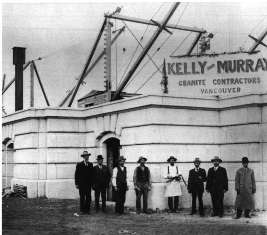
Figure 3 The recently completed granite walls of the Legislature support the contractor's sign in 1909. Allan Jeffers, the architect stands with building superintendent, John Gillespie and unidentified coworkers to his right. Steam-powered cranes in the background were used for placing stone. The doorway behind the coworkers reveals the brick backing of the stone (Glenbow Archives, NA 10428).
