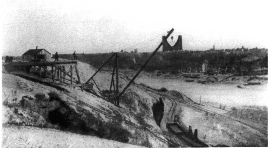
Figure 6 Siding from the Edmonton, Yukon and Pacific branch of the Canadian Northern Railway for the delivery of steel and stone for the Alberta Legislature. A five ton stiffleg derrick handed materials from the cars to a trestle and light railway on the top of the hill. To the southeast across the North Saskatchewan River the skyline of the town of Strathcona can be seen (Provincial Archives of Alberta, A 11017).
