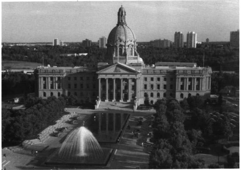
Figure 1 The Legislature from the north in 1989. The Corinthian columns of the main entrance support the provincial coat of arms on the pediment. The fountain and the reflecting pool were added in the extensive landscaping for the province’s 75 th Anniversary (Alberta Legislature Visitor Centre photograph).
