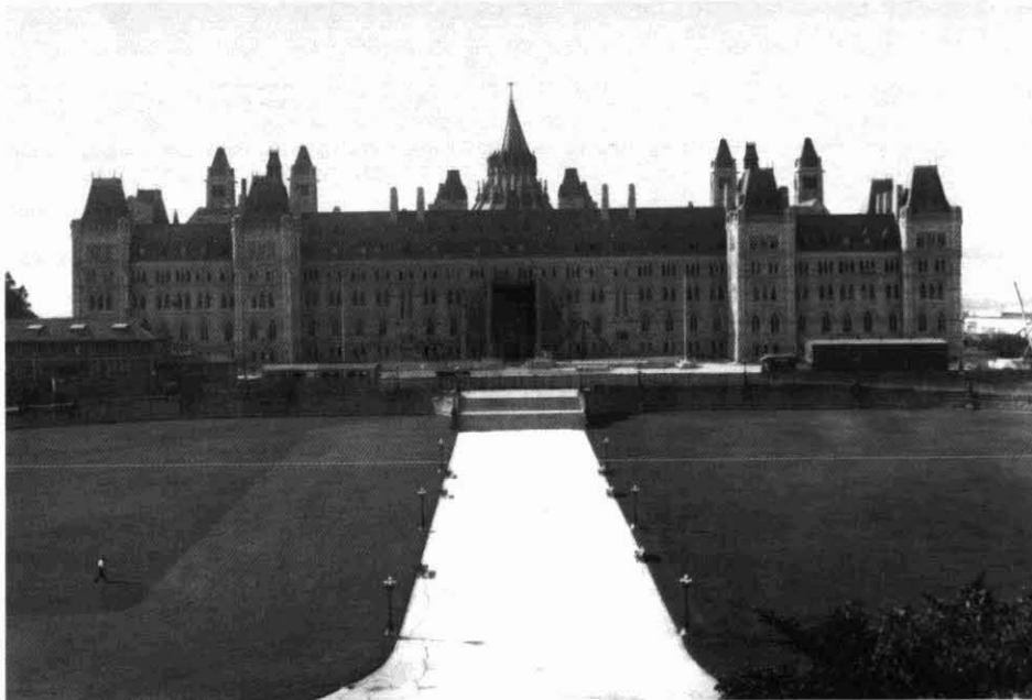
Figure 12 The nearly completed Centre Block, in 1919. Construction of the Peace Tower had not been started at this time. The stone masons' shed and the architect's site office can be seen on the left in front of the building. W.J. Topley, National Archives of Canada PA 12925.
