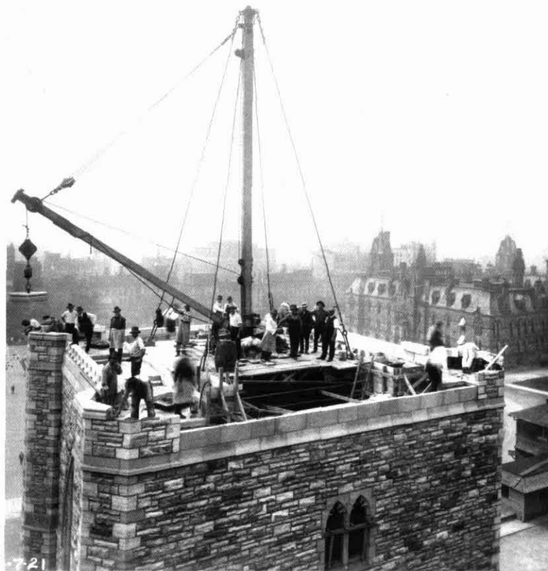
Figure 13 Stone masons at work on the Peace Tower, 4 June 1921. Note the concrete forms and the derrick used to lift and place the stone. The photo was taken from the almost completed Centre Block. The temporary building in the right foreground is the architect's office. The West Block can be seen in the background. National Archives of Canada, C38750.
