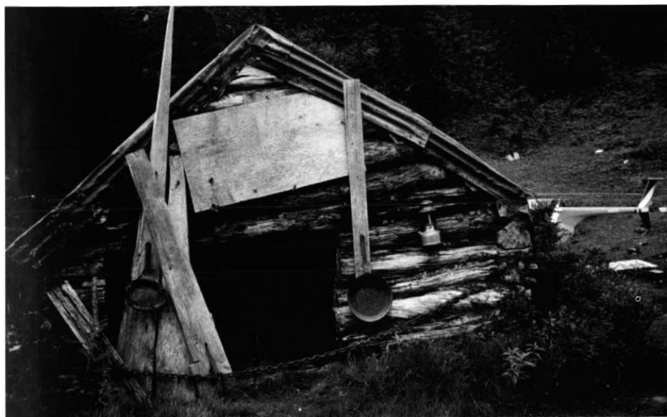
Figure 1 The old and the new: Tom MacKay's original cabin, from his early, mid-1900s prospecting programs in the Eskay Creek area, is in stark contrast to the modern, helicopter-supported program that discovered and developed the rich Eskay Creek deposit into one of the world's highest-grade gold and silver mines. Note the helicopter tail boom behind the cabin to the right. Photograph by R.G. Anderson, August 1991.
