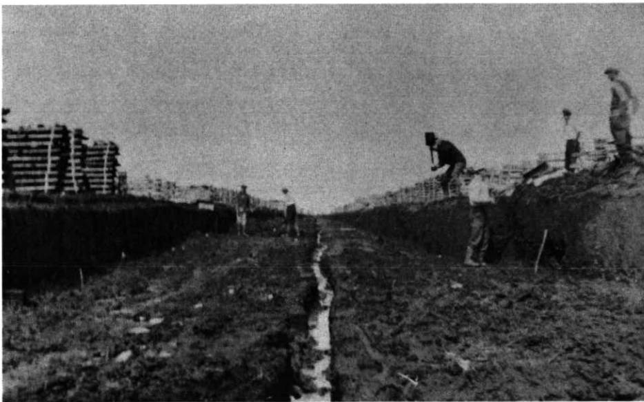
Figure 4 Hand-cutting of peat blocks in 1940s around Rivière-du-Loup, Quebec (Archives of Ministère des Ressources naturelles, Quebec).
