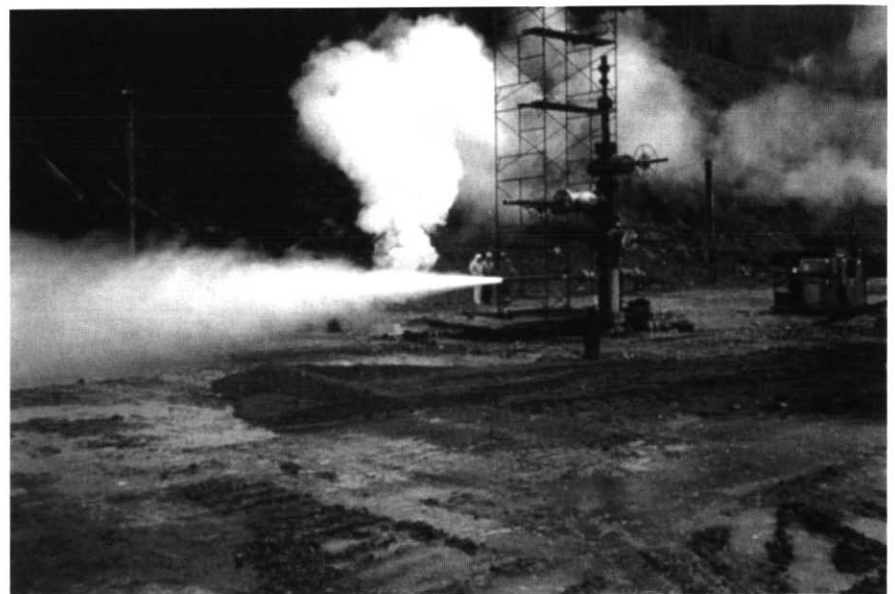
Figure 6 One of the deep exploratory wells at Mount Meager, with steam issuing from it. Three wells were drilled in 1980-1981, and a fourth well was drilled in 1995.
