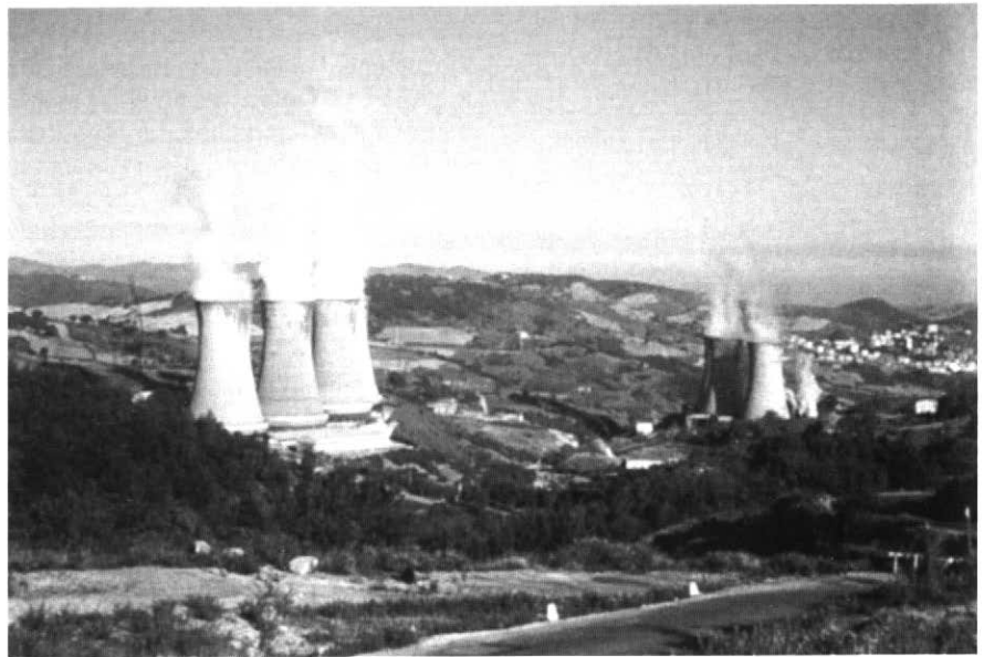
Figure 1 The cooling towers of the geothermal power stations of Larderello, Italy, where electrical power is generated from a dry-steam geothermal resource.
