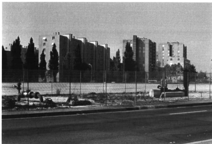
Figure 4 Apartment blocks in Paris, France, and the associated geothermal wells. Water is produced at about 50^{\circ}\text{C} to 60^{\circ}\text{C} from one well, and is taken by pipe to a heat-exchanger and heat-pump system. After use, the cooled water is returned to the reservoir by the other well. The wells are directionally drilled, so that they are about 1 km apart where they intersect the reservoir.
