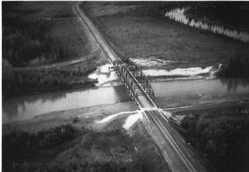
Figure 8 The Eagle River bridge, Dempster Highway, Yukon. This is a single span structure with minimal pile support in the river.
