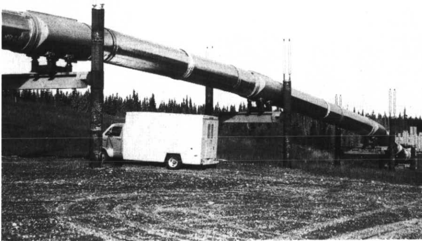
Figure 10 Trans-Alaska oil pipeline using vertical support members (VSMs) with cooling devices (fins) designed to prevent heat transfer to ice-rich, thaw-sensitive permafrost.
