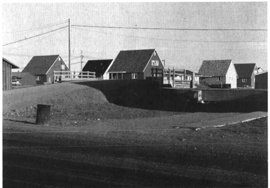
Figure 5 Inuvik, NWT, buildings are placed upon wooden piles. Services such as water and sewage are effected by a utilidor system which links each building to a central plant. (A) (top) Typical utilidor topography. (B) (bottom) Roads pass over utilidors on bridges.
