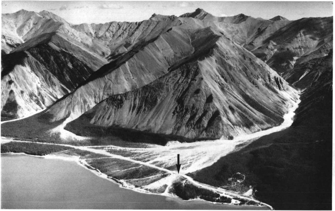
Figure 3 Oblique aerial photograph illustrating the nature of the watersheds developed in the Paleozoic carbonates of the Sentinel Ranges in the vicinity of Muncho Lake. Note active fan surface and steep bare slopes. The Alaska Highway was severed at the location indicated by the arrow (A in Figure 2) during July 1988 rainstorm. Elevation difference between Muncho Lake in foreground and peak on centre skyline is 1255 m.
