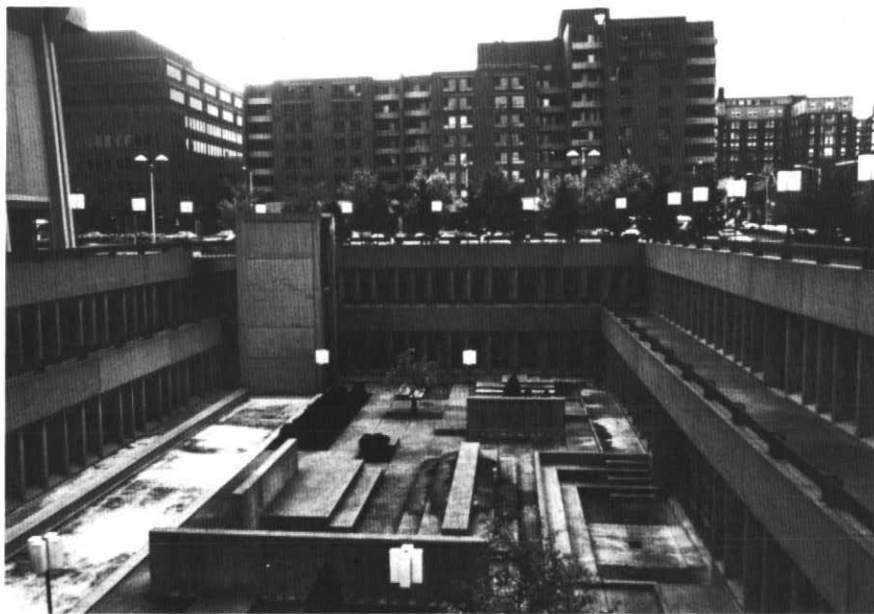
Figure 5 Quebec City's underground Music Conservatory with its central atrium, two stories deep.
