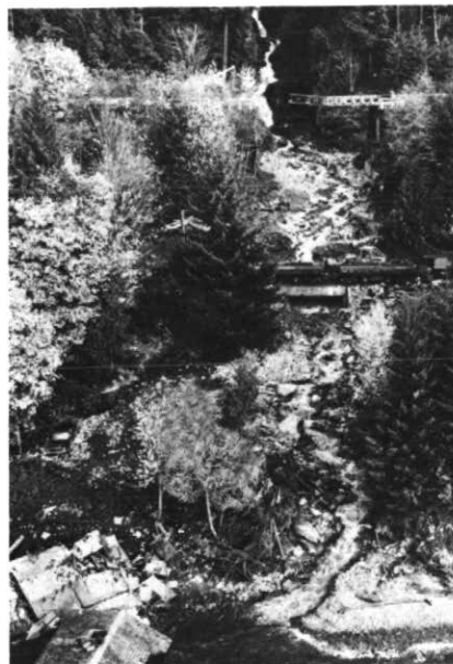
Figure 2 View of the mouth of M-Creek. Note remainders of demolished residence drifting in the sea and highway bridge under reconstruction.
