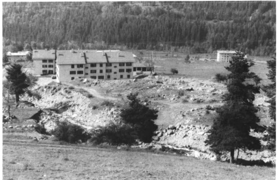
Figure 11 New apartment buildings located on blocky deposit of a historical debris flow near Briançon, France. In recent decades the forest cover of the catchment area of this torrent has improved markedly over the state it was in at
