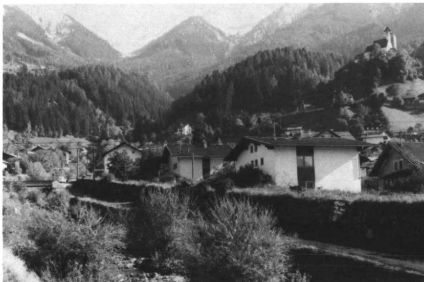
Figure 4 Elevated channel across the fan of a formerly notorious torrent that used to ravage the Medieval mining town of Schwaz, Austria. In this century, the upland debris sources have been brought under control by reforestation, check dams, and snow-avalanche fences; in
