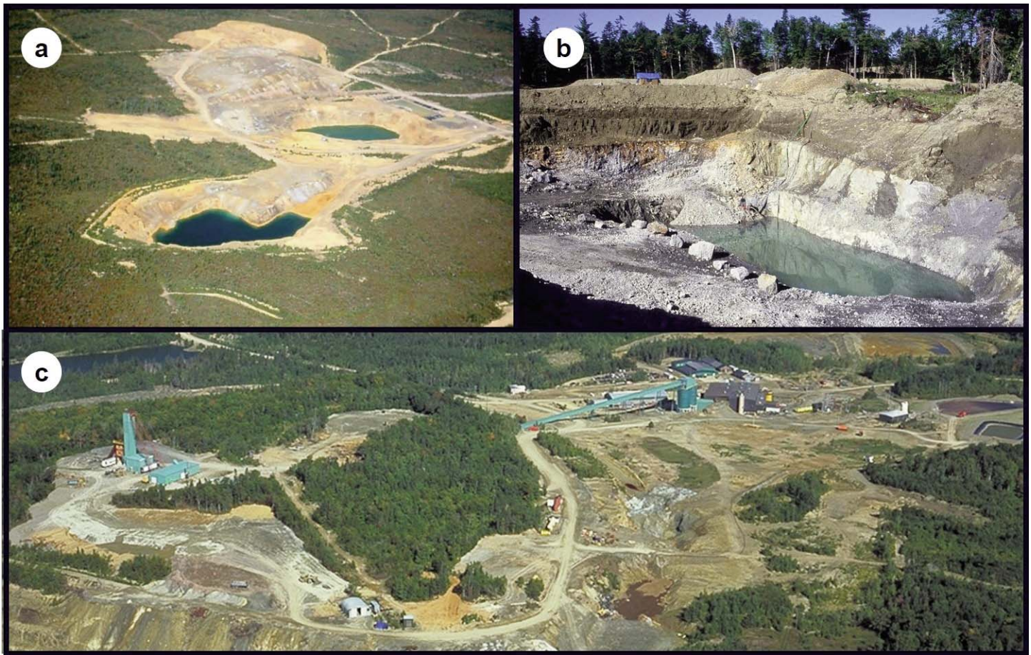
Figure 15. 1990s developments: a) aerial view looking northeast of the flooded Stratmat Boundary (foreground) and N5 (background) open pits in 1997 (New Brunswick Natural Resources and Energy Development archives); b) view looking east of the partly flooded CNE open pit in 1991 (NBNRED archives); c) aerial view looking north of the Caribou mine site in 1997 (NBNRED archives).
