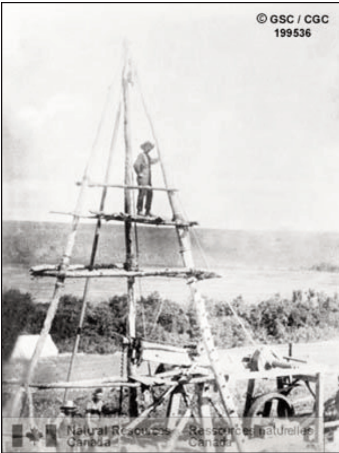
Figure 2. Example of early Geological Survey of Canada (GSC) economic geology investigations. In 1880 the GSC contracted for a number of drill holes on the southern prairies to investigate the extent of the lignite deposits exposed on the Souris River. After experiencing considerable difficulty in obtaining suitable timber for the derrick and an engine bed, this hole near Roche Percée was drilled to a depth of 295 feet. Photo Credit: A. Selwyn, second director of the GSC.
