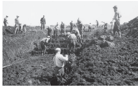
Figure 6. Photograph taken in 1940 of construction of a road through a peatland in the vicinity of St.-Ulric near Matane on the Gaspé Peninsula, Quebec. Peat was cut and removed by hand to near the mineral base. A bed of gravel was then laid down and an asphalt surface was then applied on top of the gravel. (Photograph courtesy of P. Buteau, Quebec Ministry of Natural Resources).
