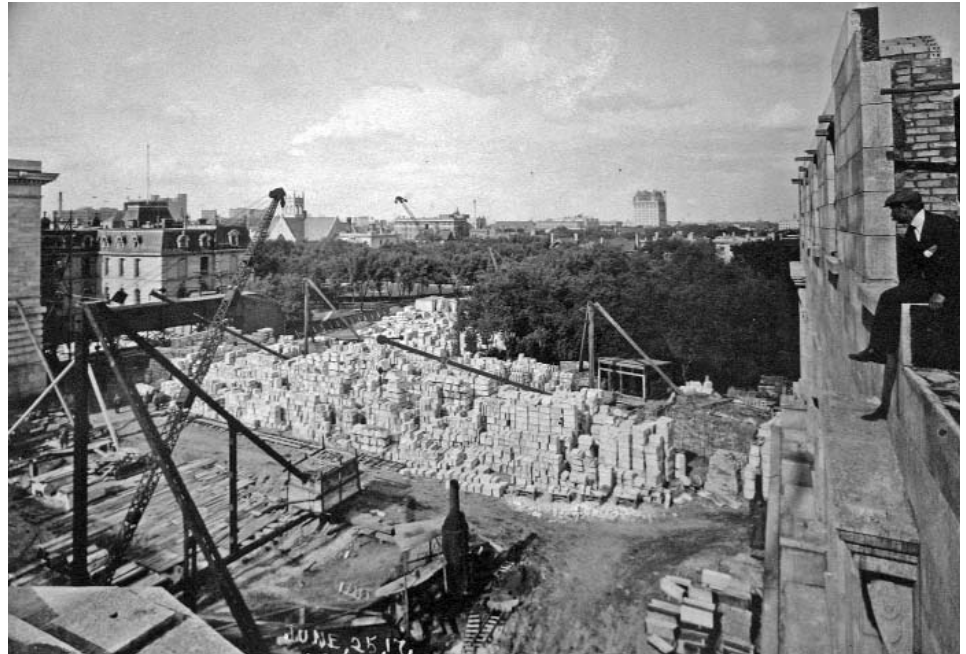
Figure 2. June 1917; an observer on the SE wing of the Legislative Building overlooks the east grounds of the building site (AM, Foote Collection 82). A brick bearing wall with Tyndall Stone facing occurs behind the observer. Blocks of Tyndall Stone are stacked in a staging area below. The old Manitoba parliament building is located on the left side of the photograph adjacent to the NE wing. The Fort Garry Hotel is the tall building in the distance.
