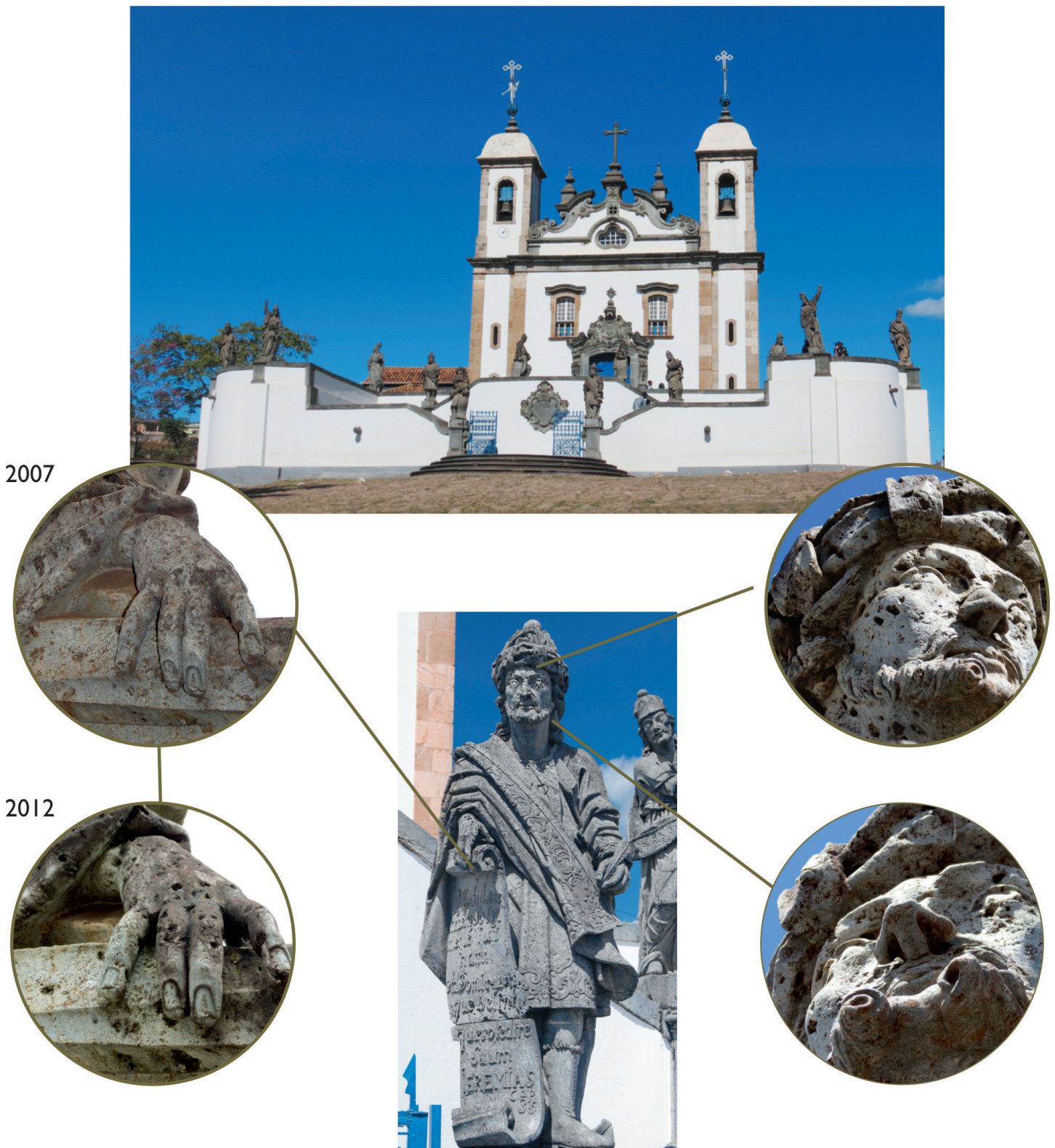
Figure 6. Deterioration of steatite (soapstone) works produced in the late 18 th century, such as those shown here in Congonhas Sanctuary, mainly caused by weak rock resistance, and by biological and anthropological factors leading to cavity or alveoli formation.
