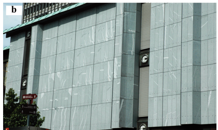
Figure 10. a) Granodiorite is used in the staircase of the Slovenian Parliament. Dark grey panels of the façade are made of cizlakite. Photo: Matjaž Zupanc. b) Maximarket department store with granodiorite façade. Photo: Miran Udovč.
