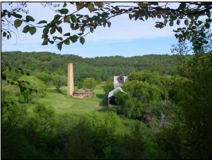
Figure 4. Historical site of the Leary brick plant near the community of Roseisle. This kiln was operational from 1900 to 1950, utilizing shale from Morden Member of the Carlile Formation.
