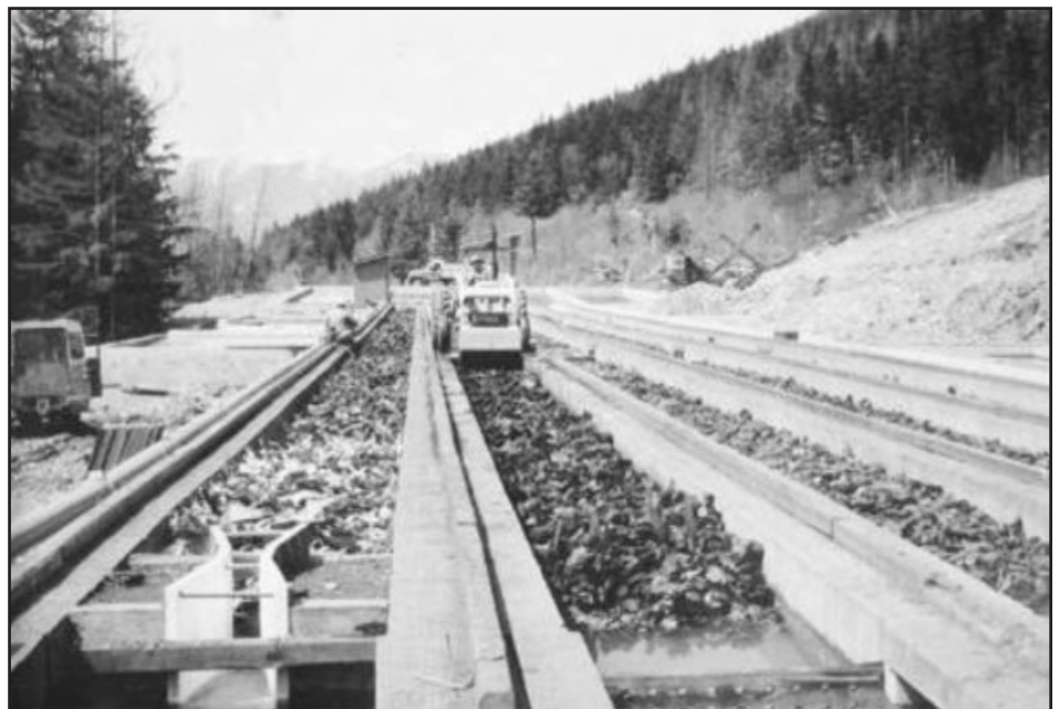
Figure 21. Copper precipitation plant launders, Mount Sheer, circa 1960. BMM Archives 13797.
