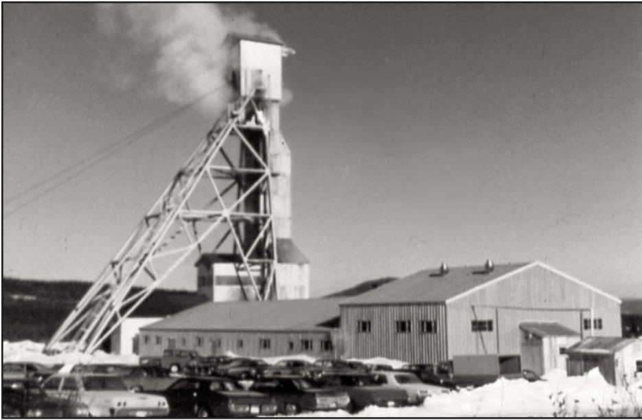
Figure 22. The MacLean Mine headframe looking north (1978). Photo courtesy of the Buchans Miners Museum.
