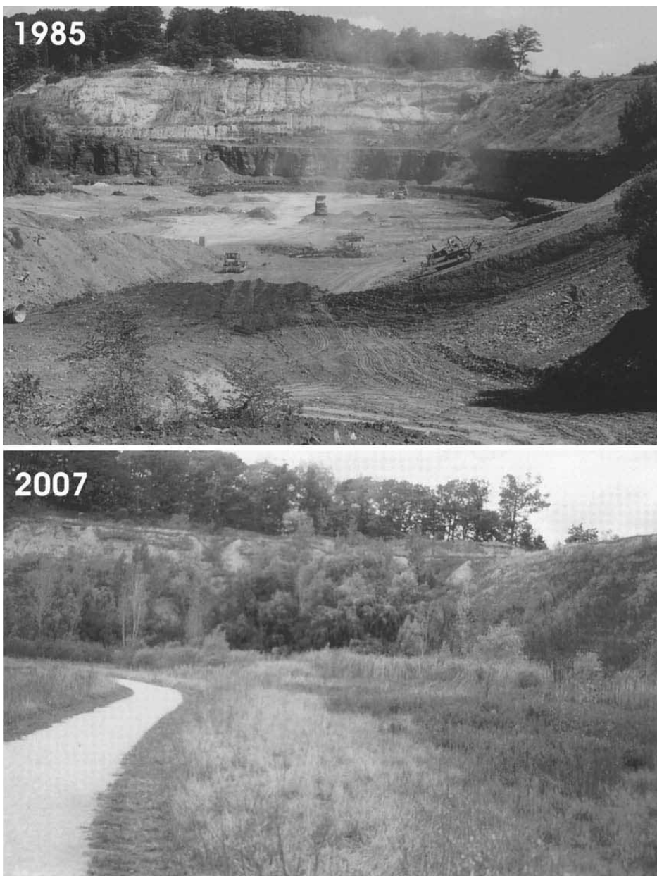
Figure 12. Don Valley Brickyard, Toronto, which produced brick from glaciolacustrine clay and Ordovician shale bedrock. Top: Don Brickyard, July 10, 1985, after purchase by Ontario government. Back-filling of the bedrock quarry is well advanced, with the north face retained for geological study. Bottom: Don Brickyard, October 14, 2007. Landscaped quarry fill and vegetative growth increasingly obscure the north face. Photos by P.F. Karrow.
