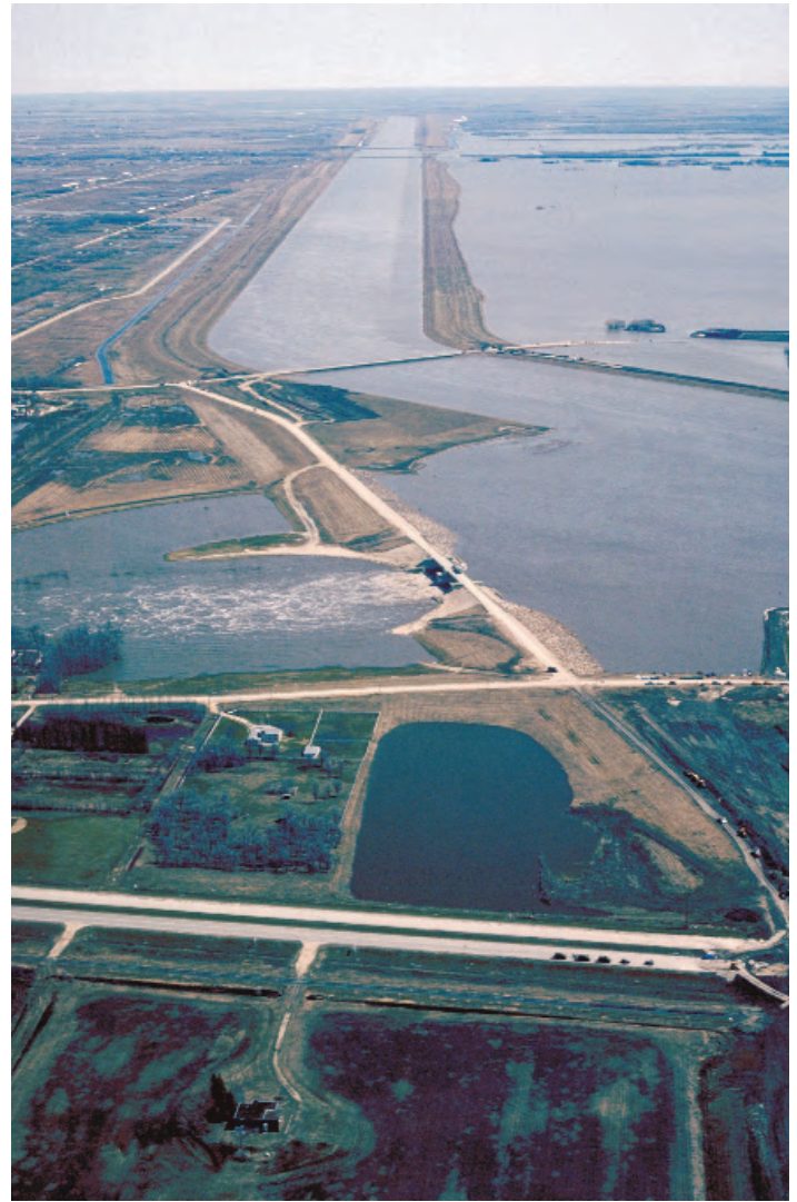
Figure 16. The Red River Floodway was built after the river flooded Winnipeg in 1951. The photograph shows the control structure at the south end of the city that diverts part of the Red River flow into the Floodway. Photo by Greg Brooks, Geological Survey of Canada.
